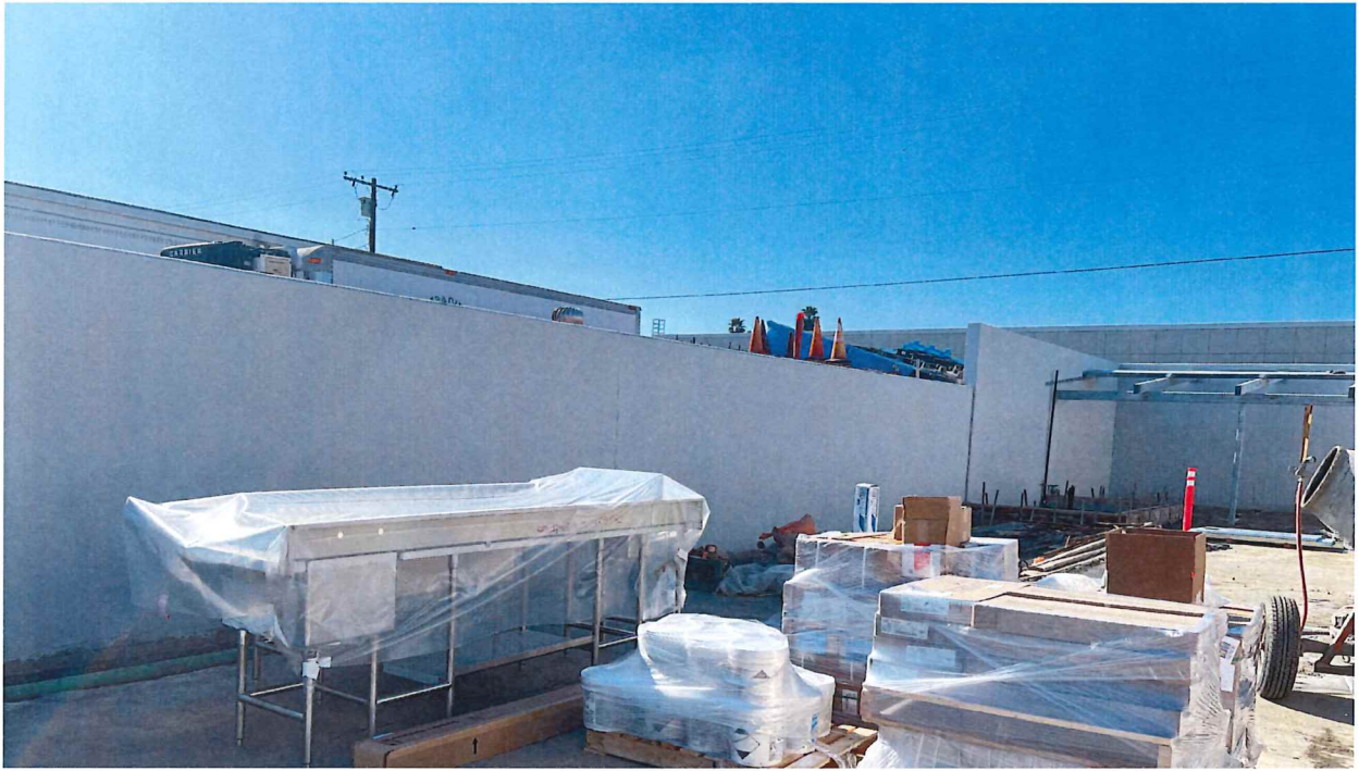
Photo: CMU wall completion
