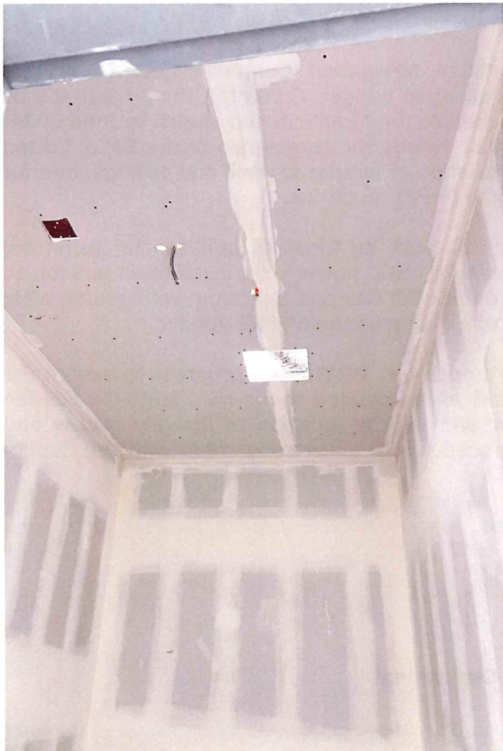
Photo: Dry wall and ceilings installed
