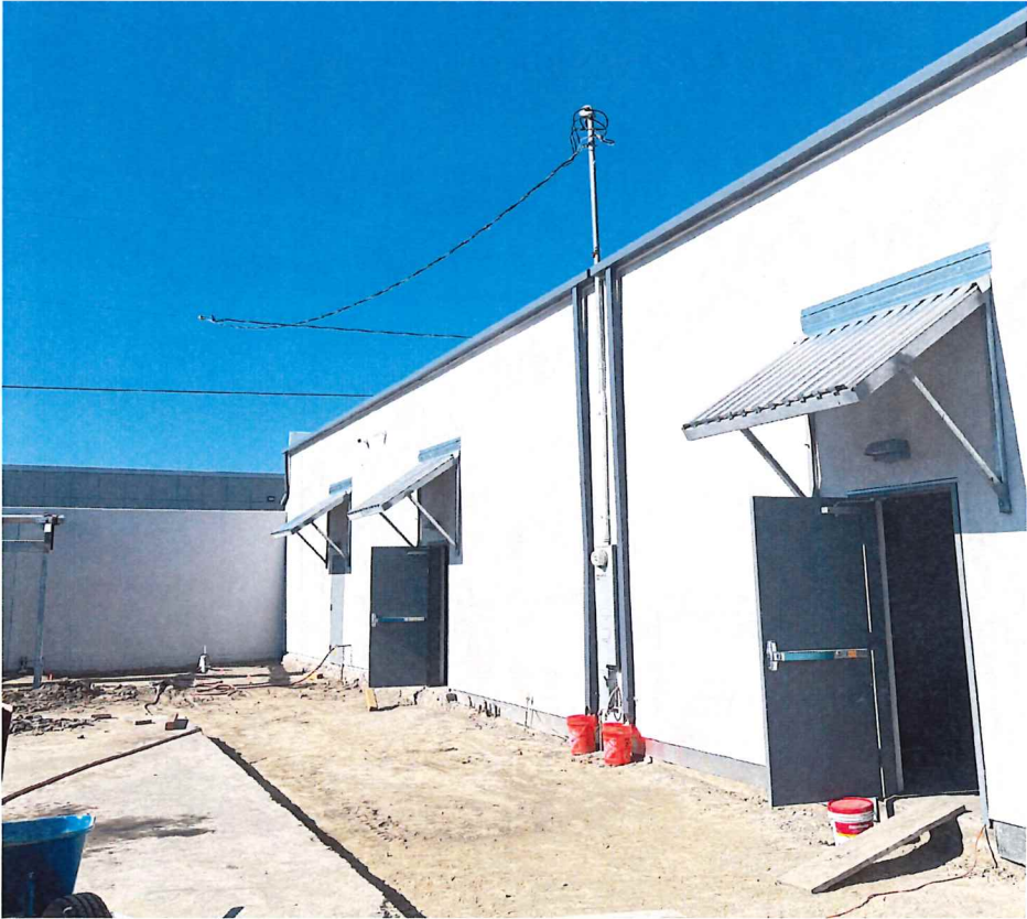
Photo: Exterior canopies installed
