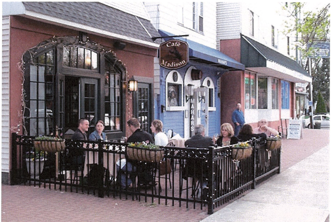
Photo 9.18-3a: Example of a fabricated wrought iron barrier.
